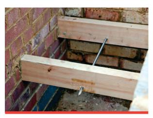
BowTie HDs installed through parallel floor joists
